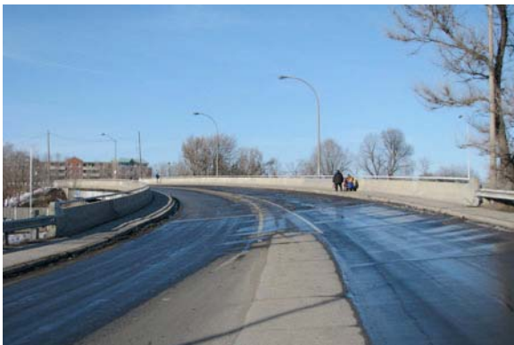
A view north across the bridge depicts one northbound and one southbound lane. Sidewalks are located on both sides of the bridge deck. The handrail system dates to 1986.
