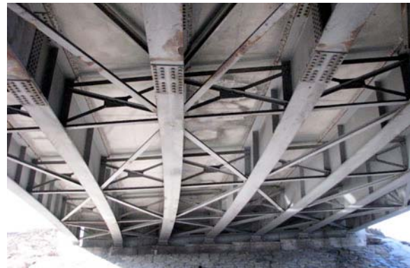
A view north through the underside of the north span shows the seven steel plate girders with cross bracing.
