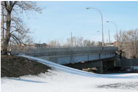
A view along the east side of the bridge illustrates the curved form of the girders and bridge deck.
