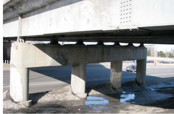
Four circular columns, each 3-ft. 6-in. in diameter, with pier cap make up the two piers.
