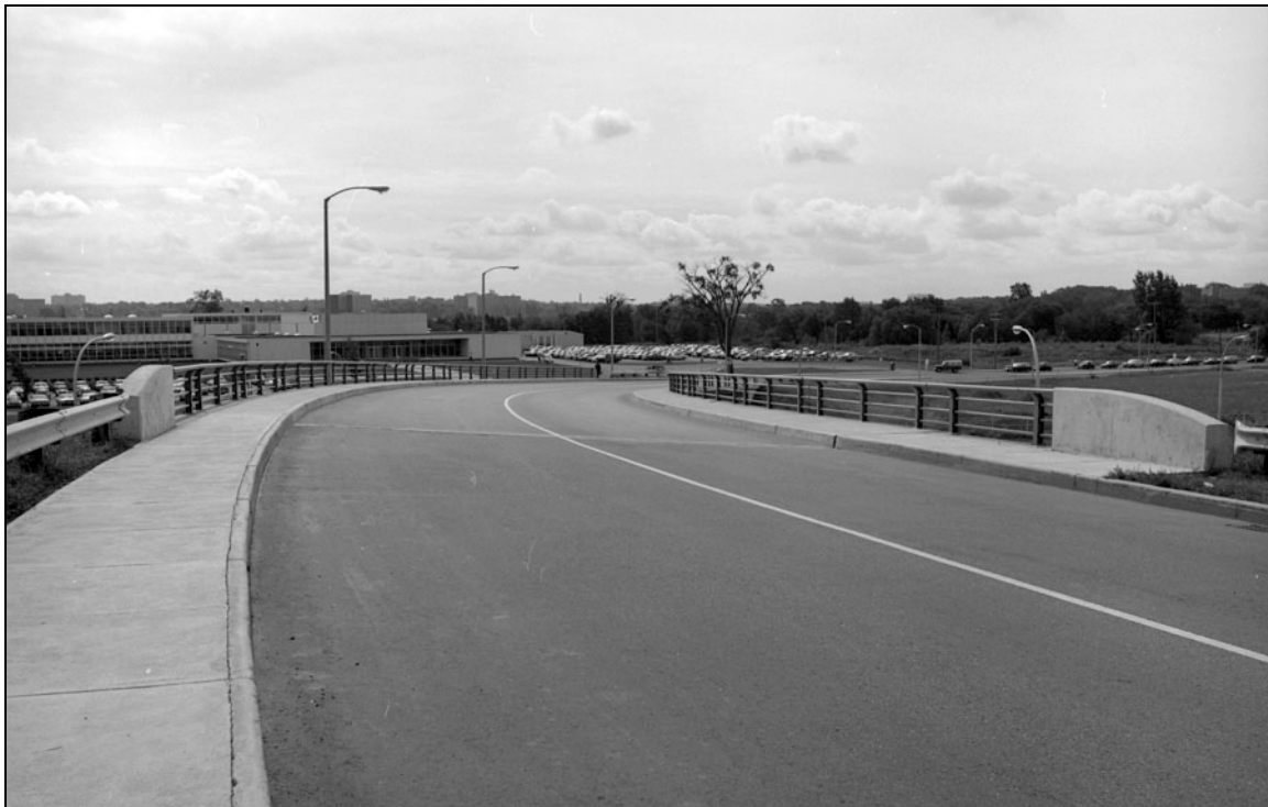
Figure 4. A view south over the bridge deck depicts the two-lane paved roadway with sidewalks, handrail system and lighting, September 1969 [AO RG14-151-4, A1302, B410835].
