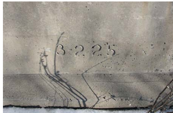
A bridge site number stamp was added to the outside of the barrier wall in the northwest and southeast corners as part of the 1986 rehabilitation work.
