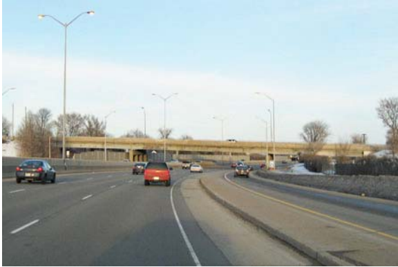
The west elevation shows the three-span, constant depth, steel plan girder underpass with perched abutments, which dates to 1965.
